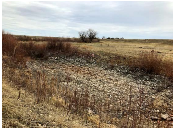
Drop structure installed to prevent head cutting of Crow Creek.
