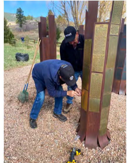
Pilot holes are drilled so the rivets fit during the placement of the plaques.
