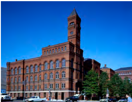
The Sidney R. Yates Federal Building - headquarters for the U.S. Forest Service.
